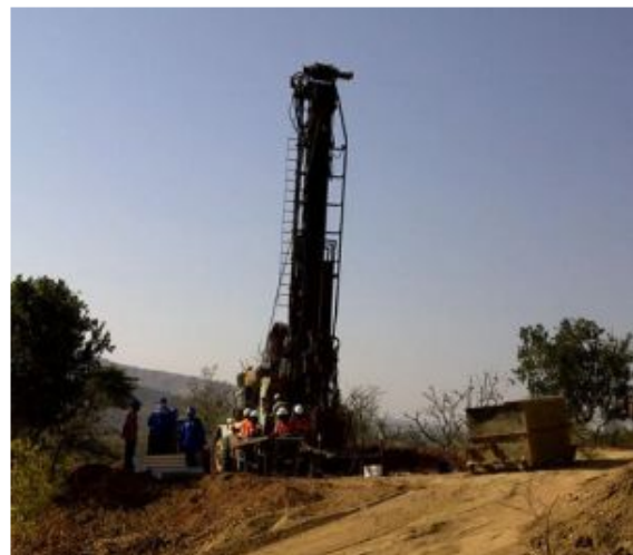
Drilling at Mkomolo
